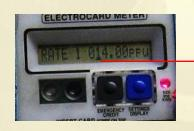
TO TO CHANGE THE PENCE PER UNIT, PRESS AND RELEASE THE GREY BUTTON (EMERGENCY CREDIT) UNTIL THE CURSER IS FLASHING UNDER THE DIGIT YOU WANT TO ALTER, WHEN THE CURSOR IS FLASHING UNDER THE CORRECT DIGIT **DO NOT RELEASE IT.** (IF YOU GO PAST THE DIGIT YOU WANT TO CHANGE JUST KEEP PRESSING THE GREY BUTTON UNTIL THE CURSOR MOVES UNDER THE DIGIT YOU WANT TO ALTER).
